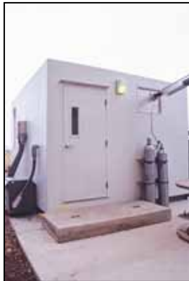
Mercury Continuous Emissions Monitoring System building at Rawhide
