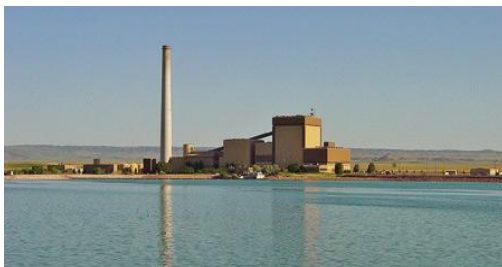
Rawhide Energy Station Wellington, CO
